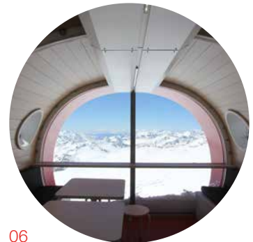
06 transparent-end; the surface is made of antiscratch acrylic sheets of the latest generation
