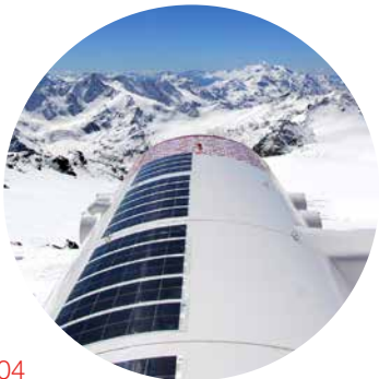
04 the photovoltaic film incorporated in the outer shell provides the energy necessary to run all the equipment
