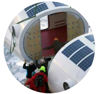
Step 3 The final assembly requires simple and quick operations to inter-connect modules and secure them onto a metal base.
